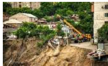
Upgrade of Municipal Infrastructure
